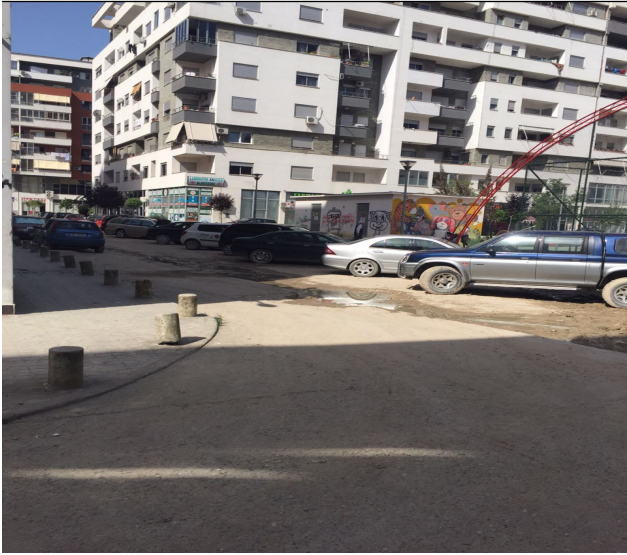
Fig.10 Segmenti ku fillon rehabilitimi i bllokut
