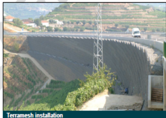
Terramesh installation
