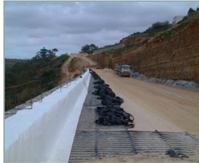
Figure 8 - Paralink in combination with Terramesh System
