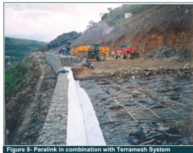
Figure 9- Paralink in combination with Terramesh System
