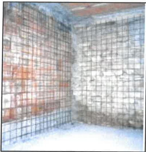
Fig. Ilustrime te perforcimit me kemishim te mureve
