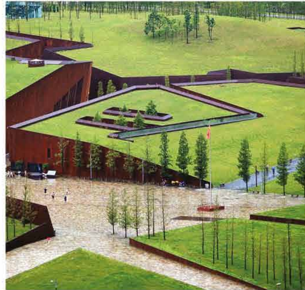
Wenchuan earthquake memorial museum. Cai yongjie. China
