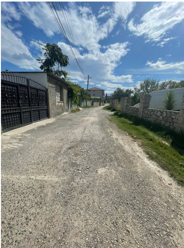
Figure 15 Rruga pa shtresa rrugore
