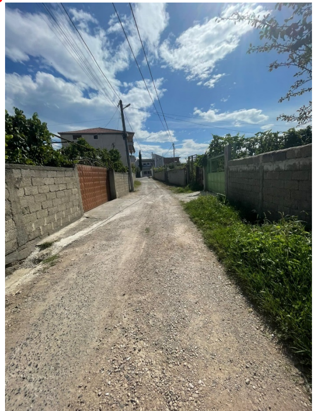
Figure 15 Rruga pa shtresa rrugore
