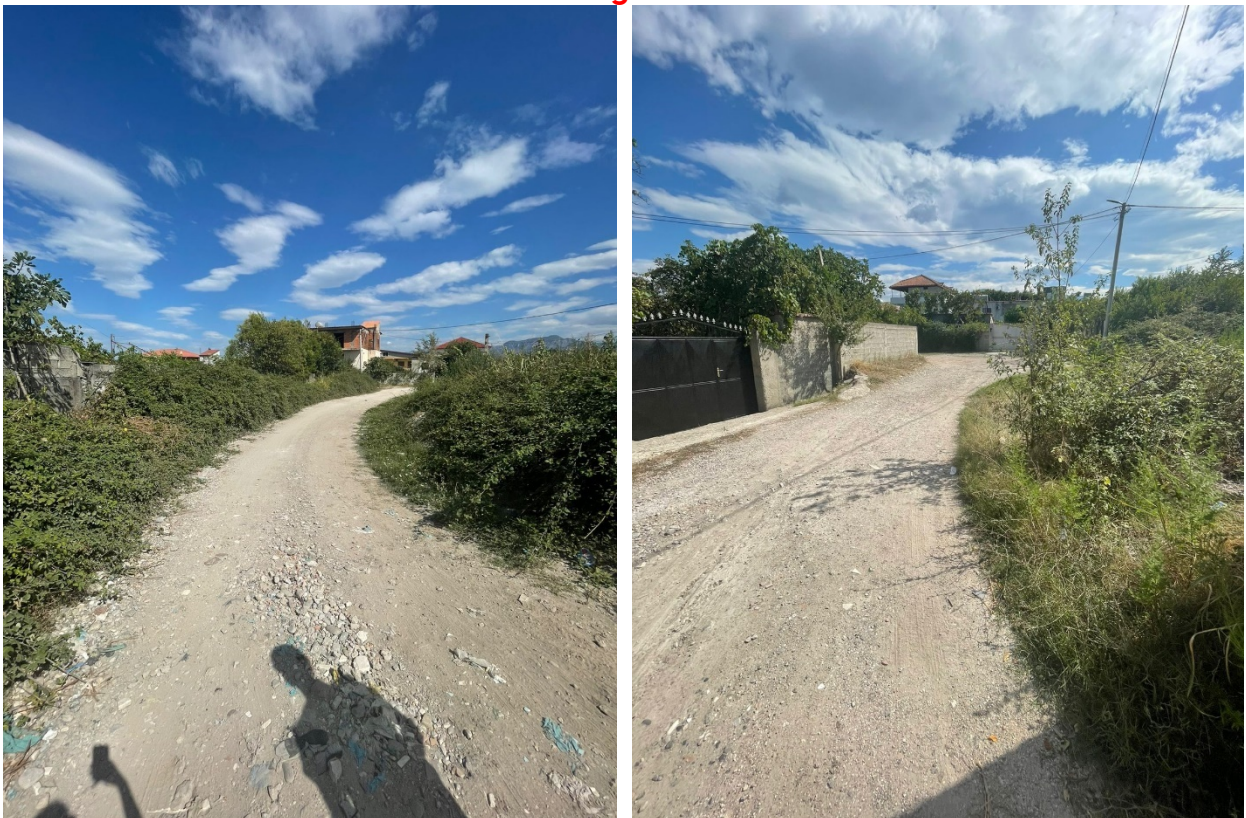
Figure 13 Dega 4- pa shtresa rrugore
