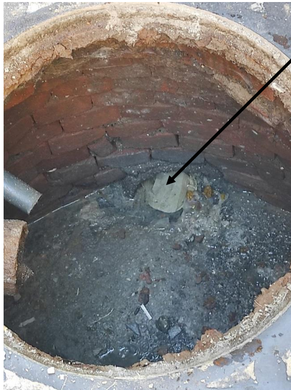
Tubacion beton DN200mm I amortizuar
