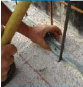
Fixing Idrostop B25 in place
