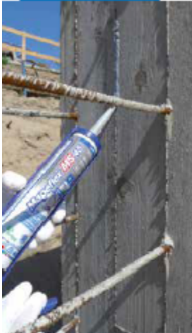
Extruding Mapeflex MS45 prior to applying Idrostop Soft in second pours
